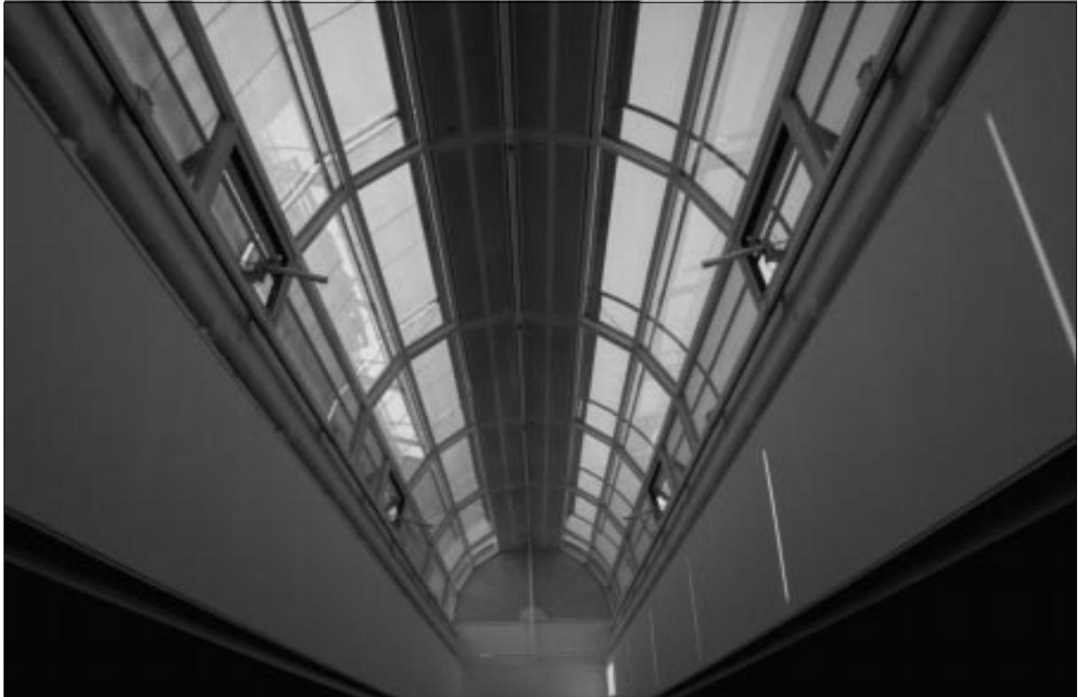
**Figure 7: Skylights in the arcade rooms. Solar protection is external fabric shading, which can be seen to the left in the picture.**
