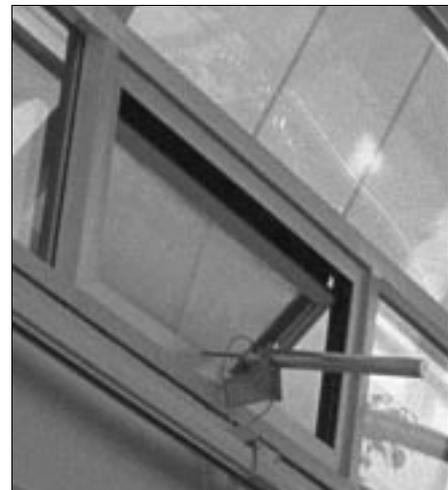
**Figure 8: The ventilation openings in the skylights in the arcade rooms are automatically controlled through a number of temperature sensors positioned in the upper part of the arcade room.**
