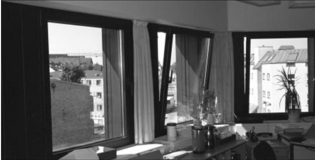
**Figure 5: In the offices there are manually operated multi-position windows, the so-called tilt and turn windows.**
